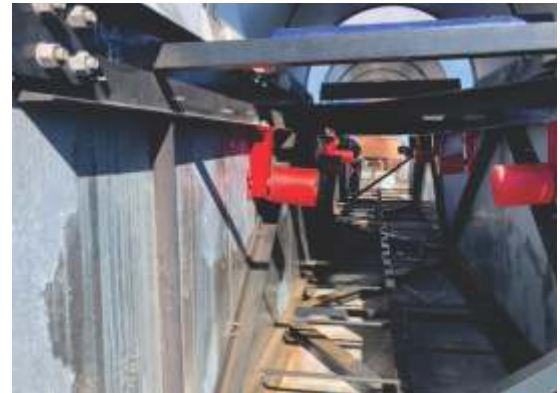
ASGCO® Stub Idler installed at a coal prep plant.
